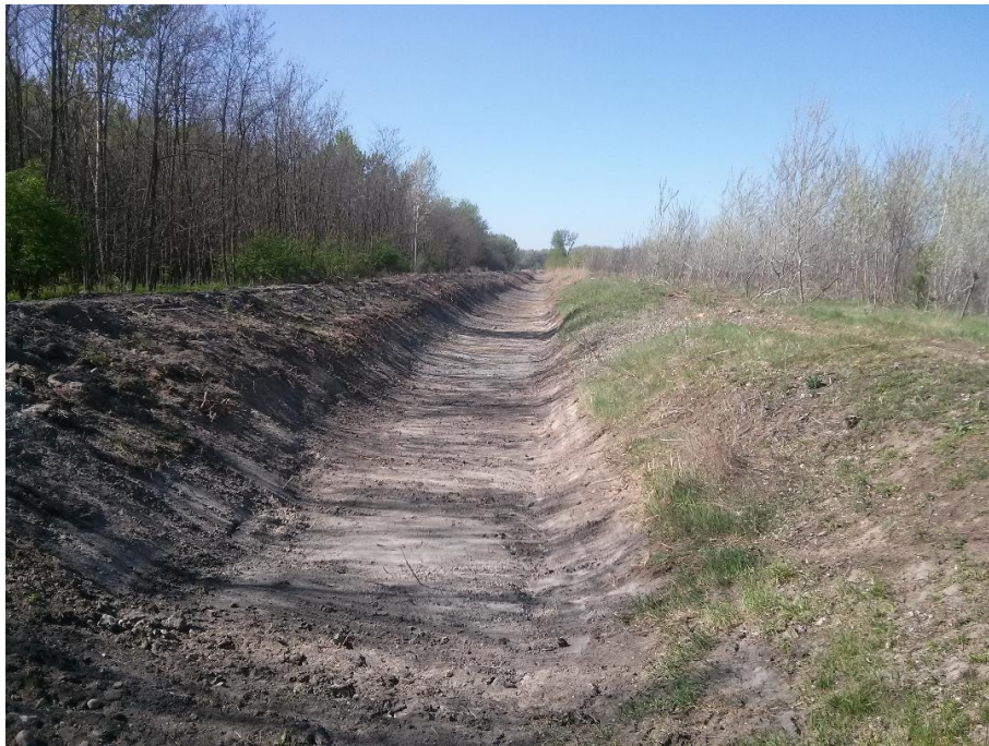
Figure 5: Unnecessarily deepened canal near Bodoglár. The attitude of the Water Management now threatens the water resources needed for forestry and agriculture.
